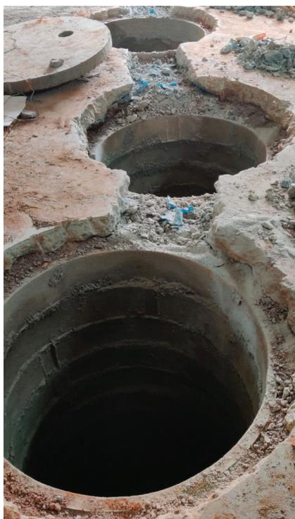
Groundwater recharge pits allow rainwater to refill borehole wells that supply water to residents in Bengaluru. Credit: Ganesh Shanbhag
