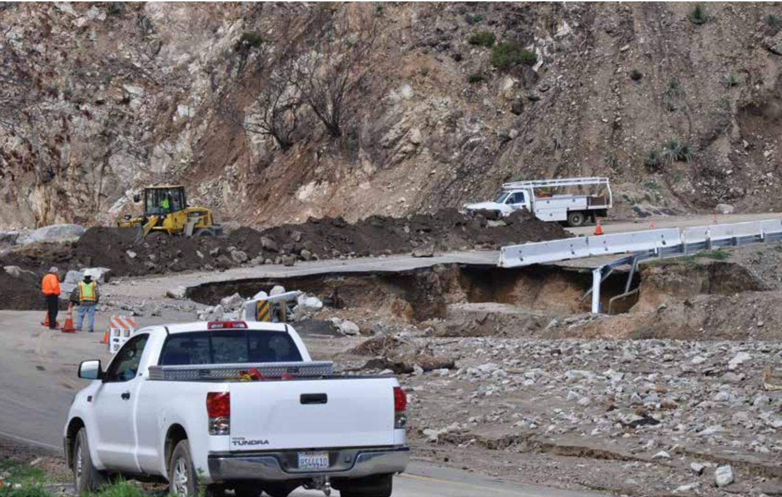
Debris flows from heavy rain after the 2009 Station Fire damaged part of the Angeles Crest Highway in Southern California. Credit: Jason Kean/ U.S. Geological Survey
