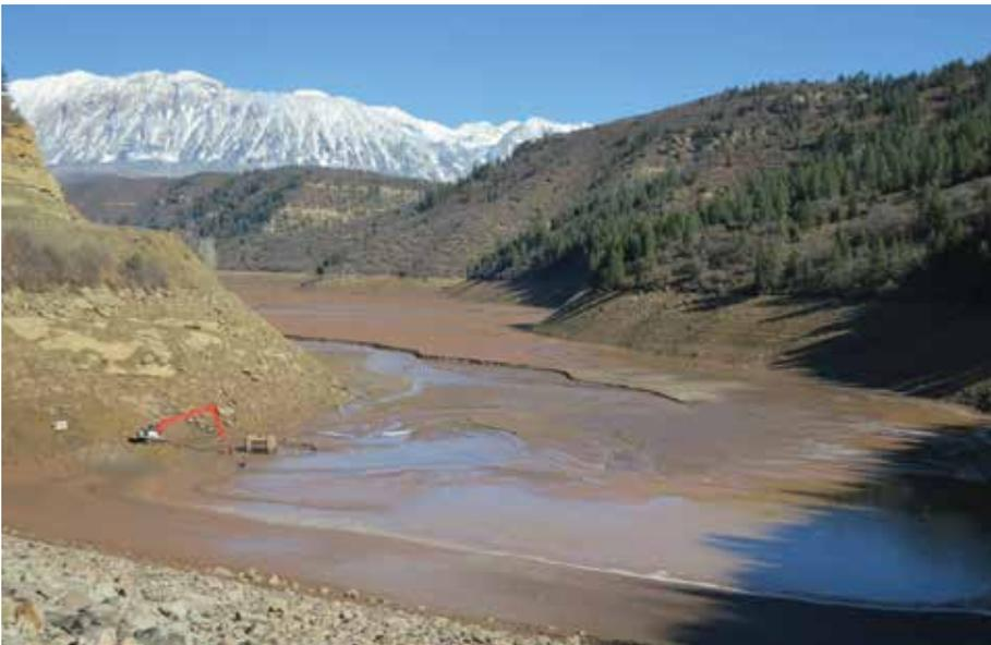
Paonia Reservoir in northwestern Colorado, seen here in 2014, reached the end of its sediment design life after 50 years when the outlet (the boxlike structure to the right of the excavator), located at the top of a 21-meter tower, became clogged with sediment. Credit: U.S. Bureau of Reclamation
